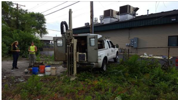
Photograph 7. A&W drilling Boring 1-1-2, view to the southeast
