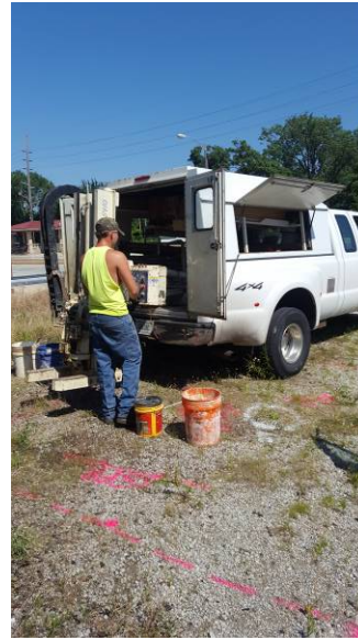
Photograph 2. A&W preparing to drill Boring B-1-1-1, view to the west
