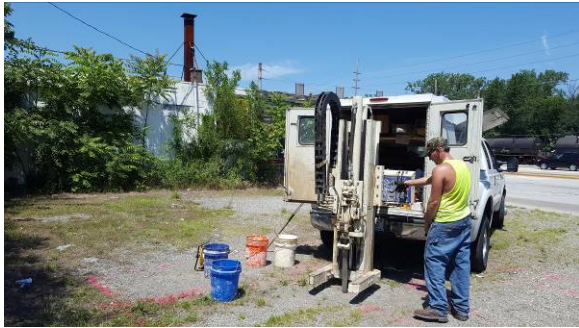
Photograph 1. A&W drilling Boring B-1-1-3, view to the northwest
