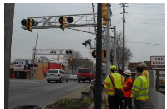
No railroad crossing signs exist for pedestrians or vehicles; Signal coordination improvements are needed
