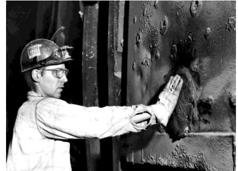
Steel worker Homer Farley of Gary operates a furnace. July 14, 1959. Tribune archives.
