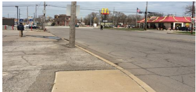
Sidewalks and driveways become one pavement surface with no delineation for non-motorized users.
