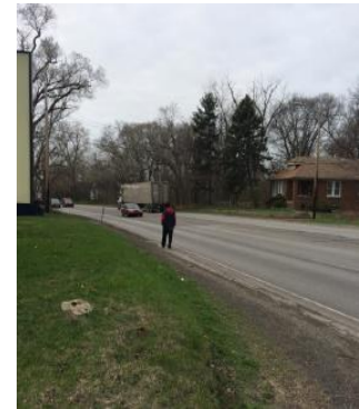
No sidewalk present; pedestrians and bicyclists use shoulder along US 20
