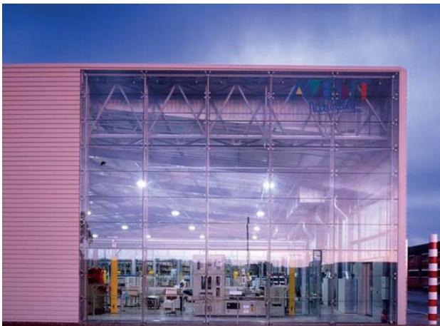
Transparency in industrial buildings can showcase activities and contribute to the high-tech character of North San José.
