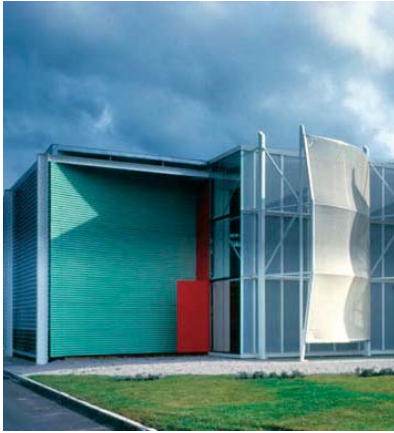
Color variations, architectural modulations, and shading devices can reduce the perceived scale of large buildings.
